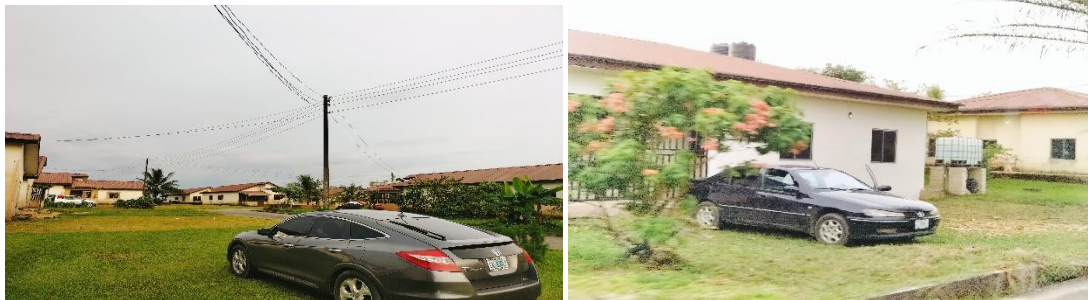
Fig. 5. Undefined Landscape and parking space pattern in the Estate. Source: Author's fieldwork, 2022.
